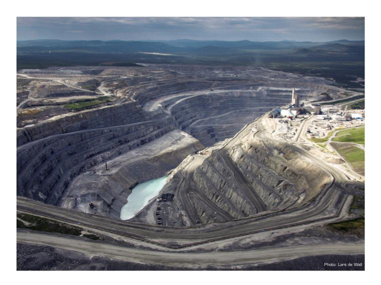
ATIK, SITUATED OUTSIDE the town of Gällivare in the very north of Sweden, is Sweden's largest copper mine. Aitik is also the most efficient open pit copper mine in the world. The deposit consists of chalcopyrite and pyrite yielding copper, gold and silver. Approximately 40 Mtonnes of ore is mined and concentrated here every year. The open pit is 3 km long, 1.1 km wide and 450 meters deep – so far.
